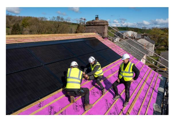
Rear elevation with 20 panel layout, maximum achievable on roof.
